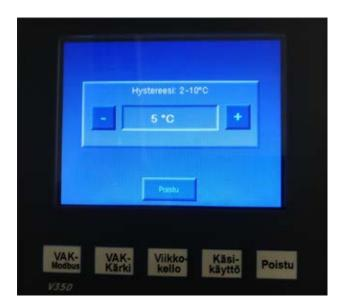
The hysteresis value can be adjusted between 2-10°C (factory setting 5°C). The hysteresis setting affects the control of the desired temperature.
